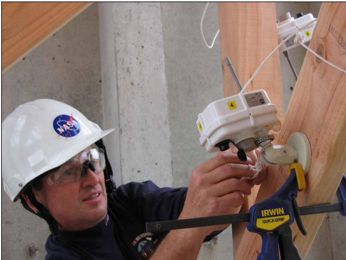
Figure 6: Pods are attached to shoring.
